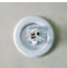
Sidewall Sprinkler
